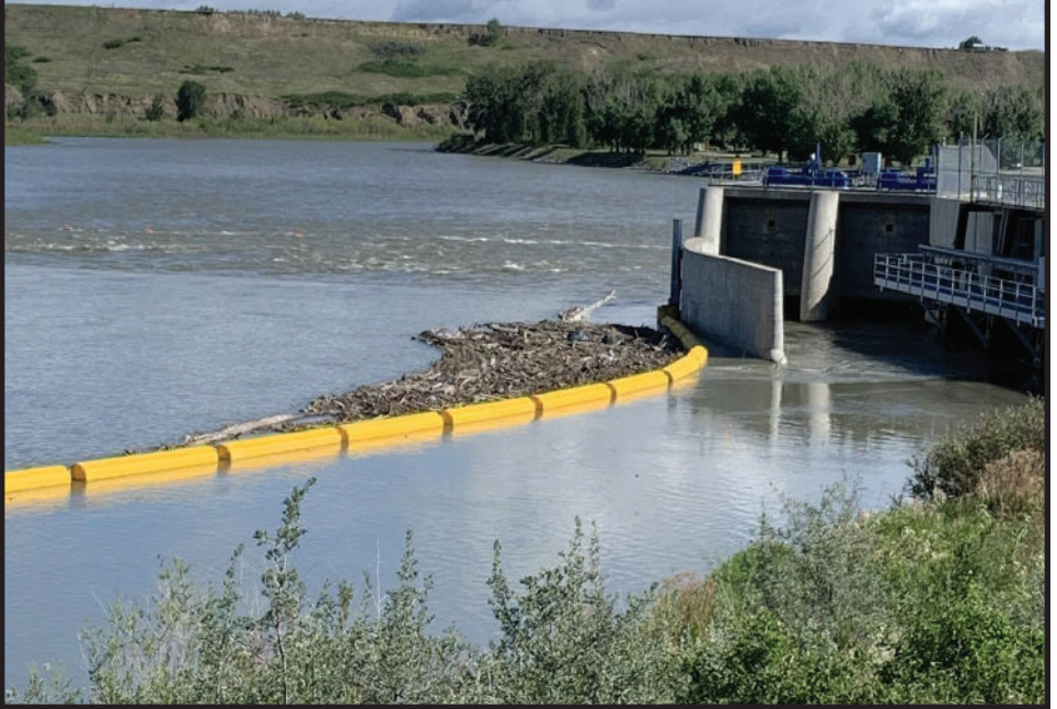
Carseland Weir Trash Boom
