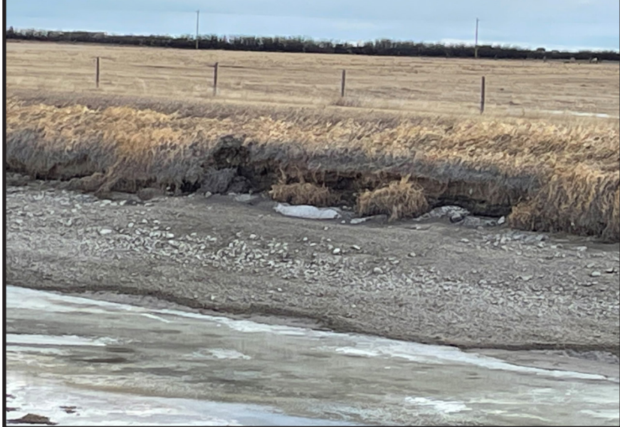
Main Canal Sloughing below Drop #3
