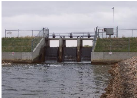
Expanse Coulee Check-Main Canal
